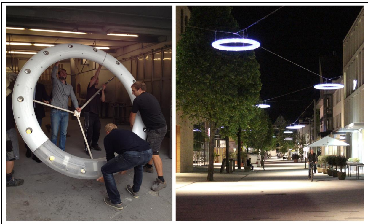
Figure 5. The semi-transparent torso-shaped luminaries specially developed for the Bahnhofstrasse in Böblingen: testing of different shell materials with the manufacturer (left) and luminaries suspended in the public space (right).
