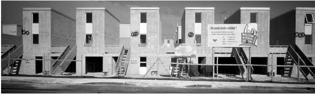
Figure 1. Elemental, Quinta Monroy , Chile, 2003. The original units built by Elemental, which are designed to be added onto by the residents.
